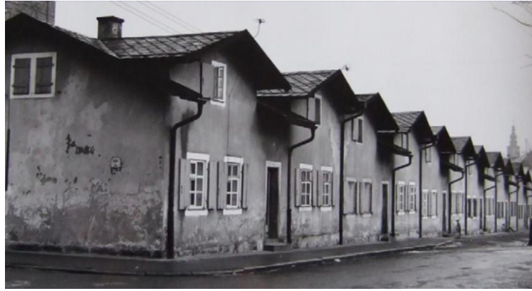
Figure 15: Borg Company Housing Estate, Bayreuth, Germany.
